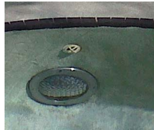
ABOVE- Skimmer equalizer without approved cover.
